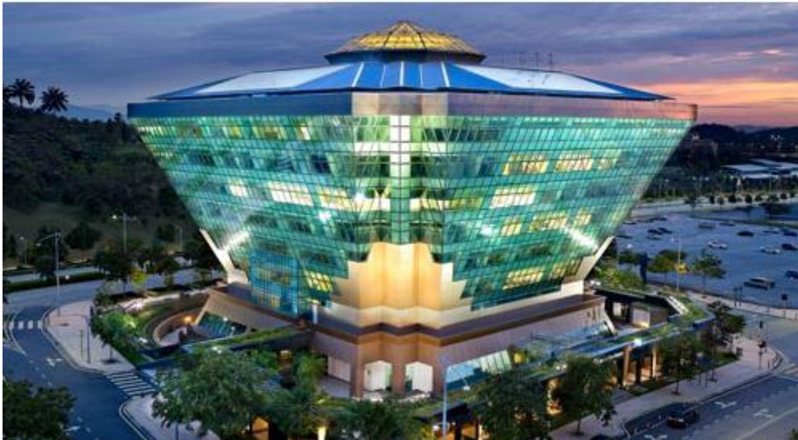
Exterior view of the building
